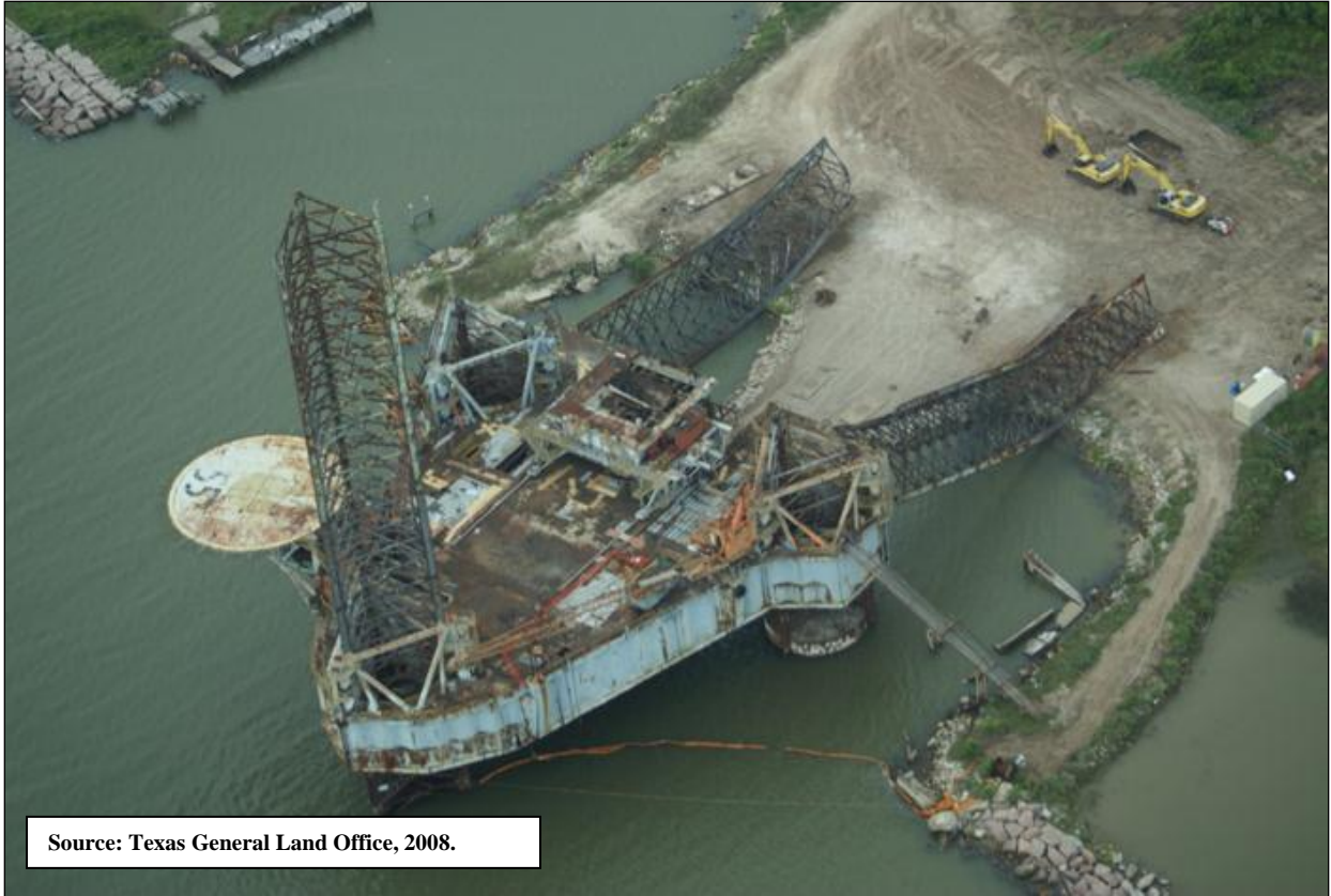
Figure A.29. The dead-stacked jackup rig Zeus being dismantled in Freeport, Texas.
