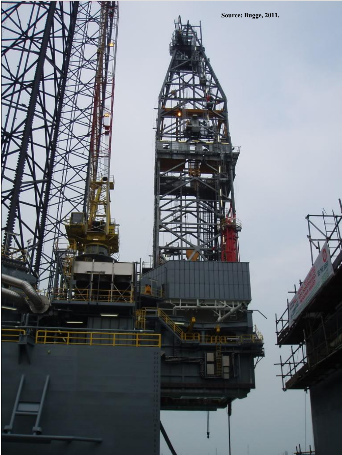
Figure J.4. A derrick and cantilever on a jackup rig.
