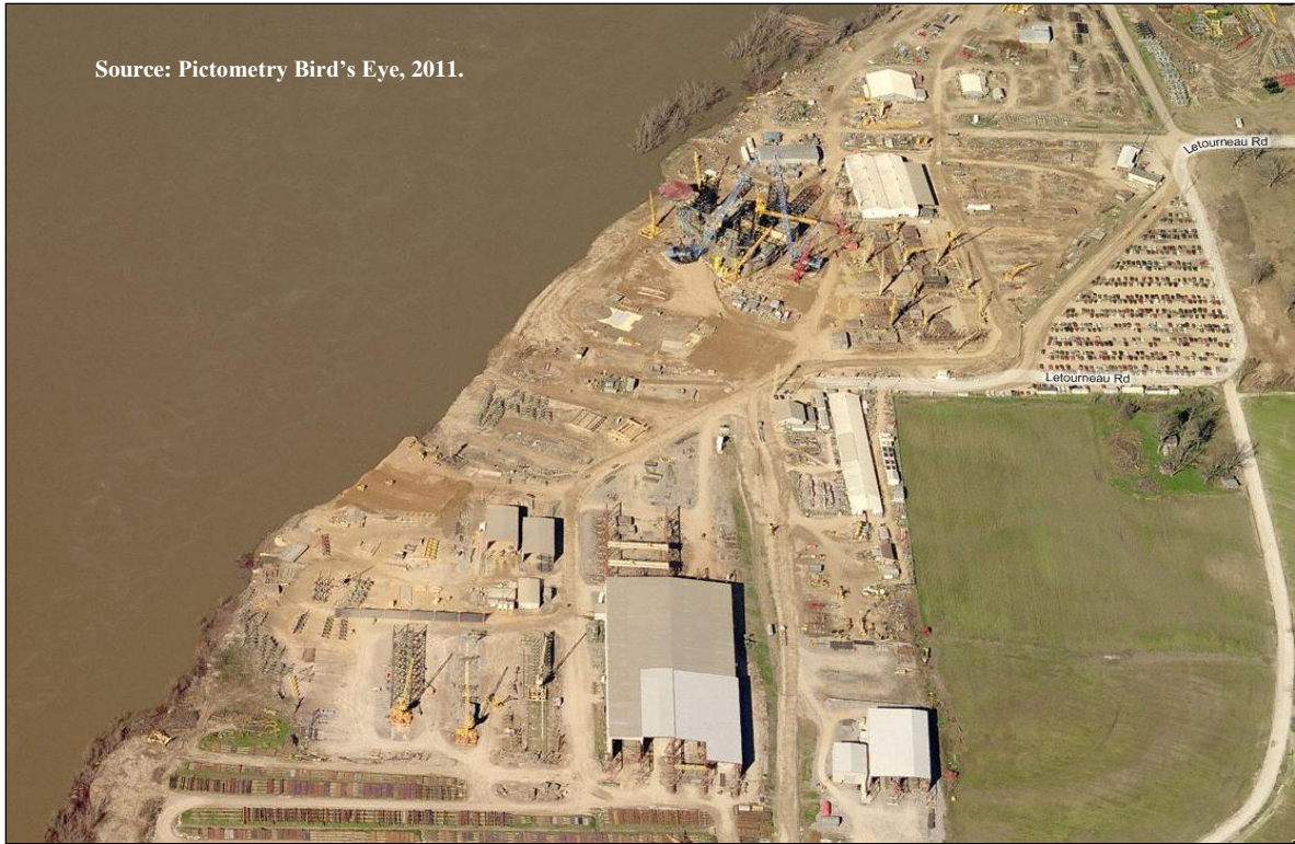
Figure G.8. The LeTourneau Vicksburg, Mississippi shipyard.
