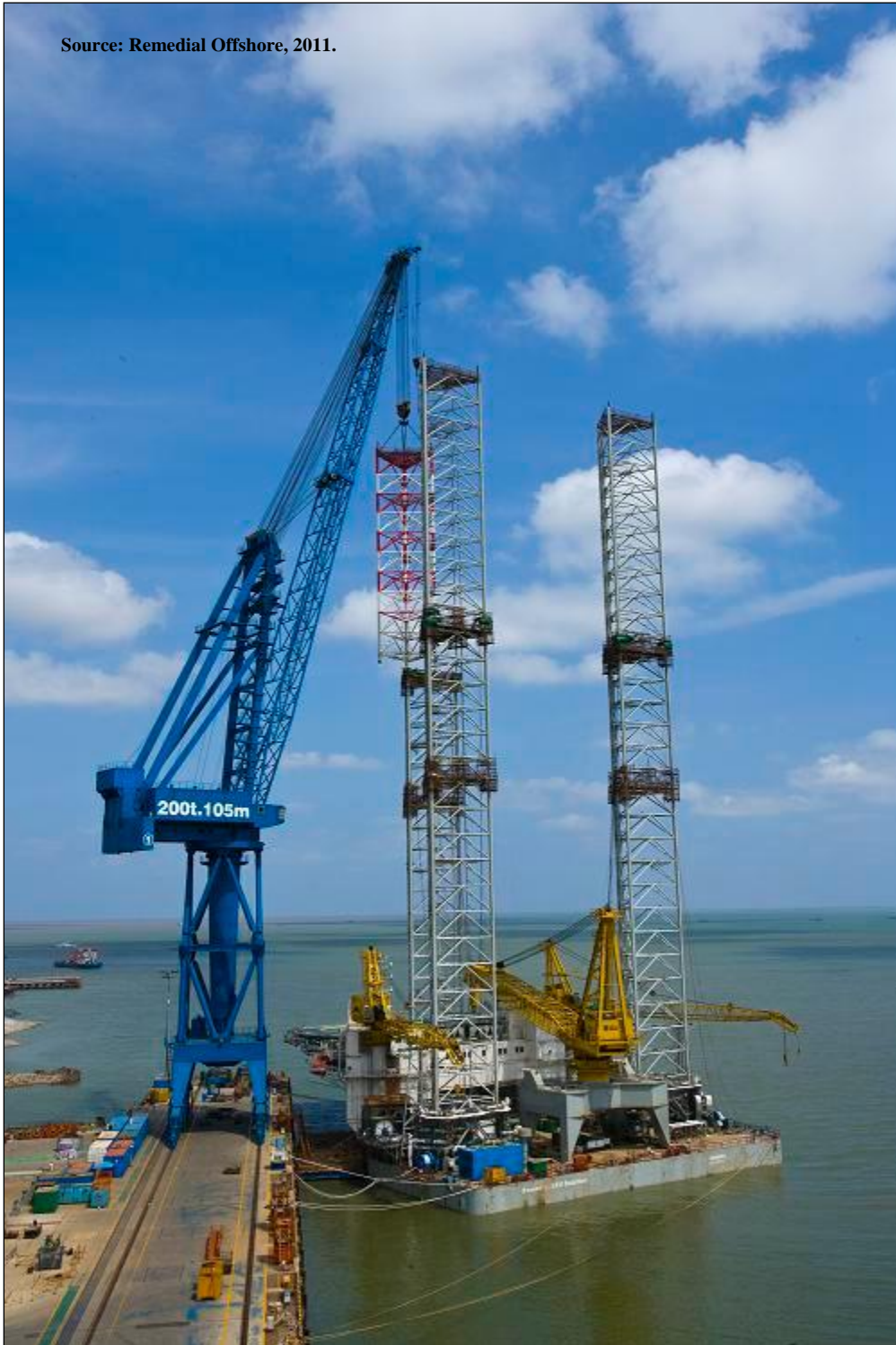
Figure I.9. Construction of F&G Super M2; top section of leg installed.
