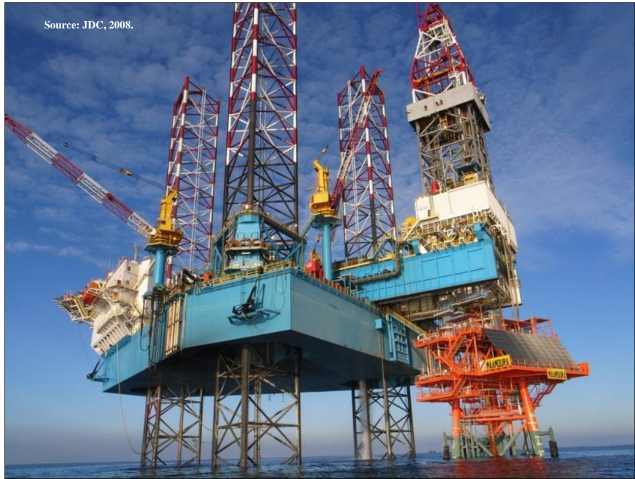
Figure H.10. Cantilever drilling rig operating over a fixed platform.
